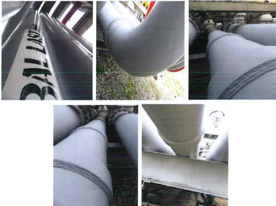
Photo2: Ballast line still in good condition observed
